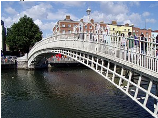
Liffey Bridge / Ha'penny Bridge
